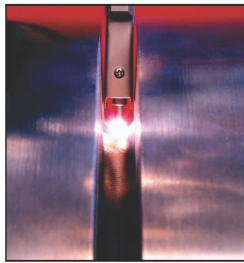
Cutting Edge Narrow-Groove Pipe Welding Technology
