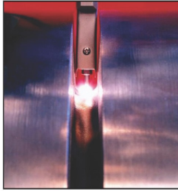
Cutting Edge Narrow-Groove Pipe Welding Technology
