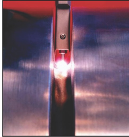
Cutting Edge Narrow-Groove Pipe Welding Technology
