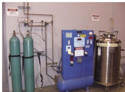
**Photo 5:** Gas supplies and controllers outside the weld lab; pure argon is used for orbital welding whereas for manual welding, argon from a cryogenic dewar is mixed with hydrogen (2%) from a gas cylinder using a mass flow controller. Gas is piped to each weld station for purging during welding.
